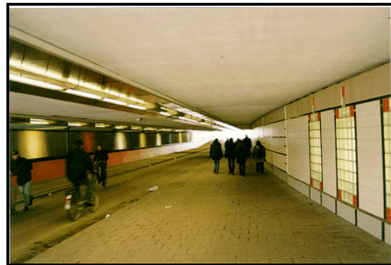
Bicycle/ pedestrian tunnel Utrecht Photo: SWOV, Institute for Road Safety Research, A. Vis
