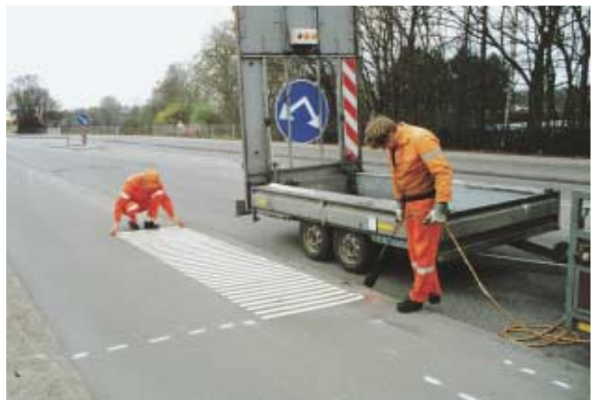
Two men for two hours and the marking of a bus stop is finished.
