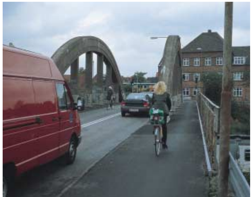
Cramped space on the old bridge over the railway in Næstved.
