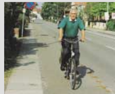
Separated cycle-footway is useable at low cyclist and pedestrian volumes.
