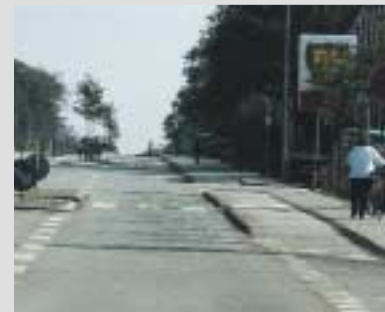
The Danish cycle track gives a good separation between road users.
