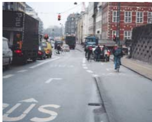
Downhill – truncated cycle track.
