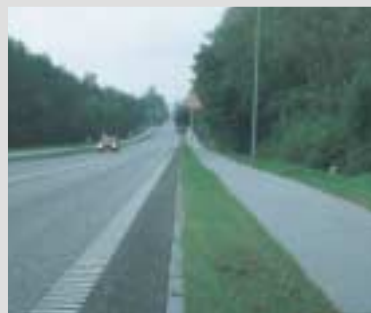
A cycle track with dividing verge is a fine solution on highways.
