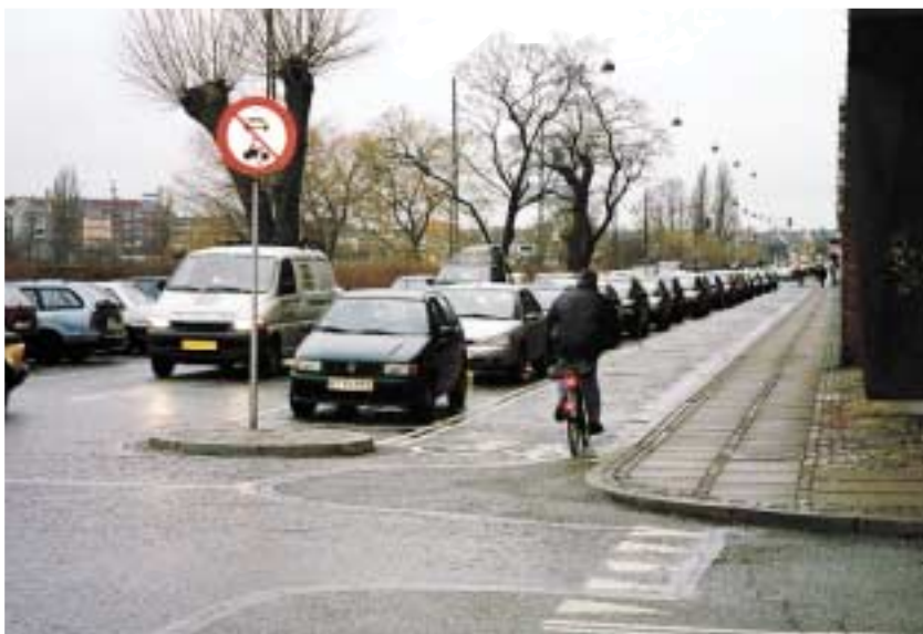
The traffic island prevents parking close to the junction.
