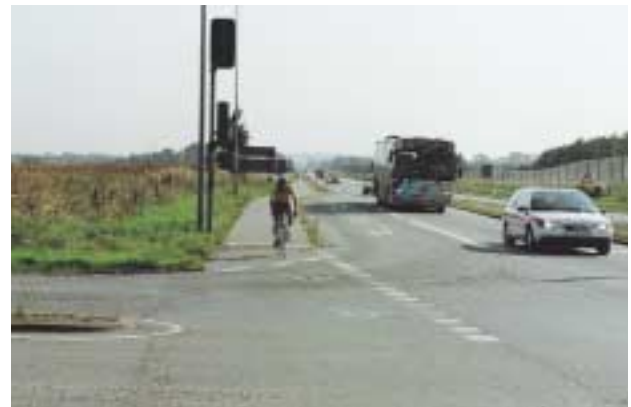
The dividing verge should end 20-40 metres before the junction in order to increase cyclists' visibility.
