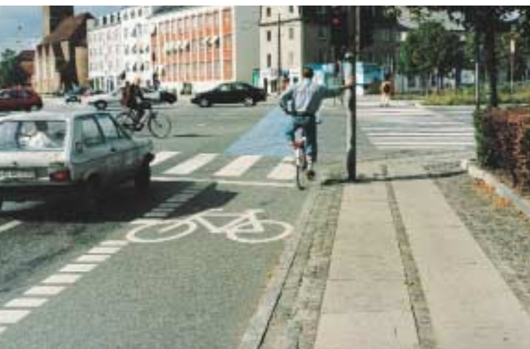
A good profiled stripe. Staggered stop lines should have been established.
