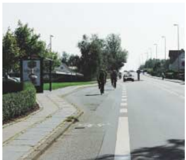
A broken edge line next to the bus bay is missing.
