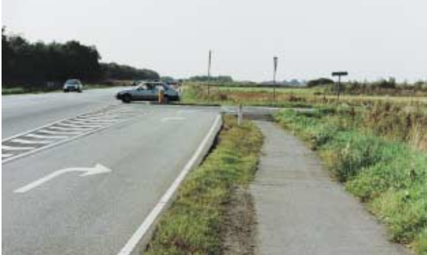
Interrupted cycle track - the dividing verge should not be there.
