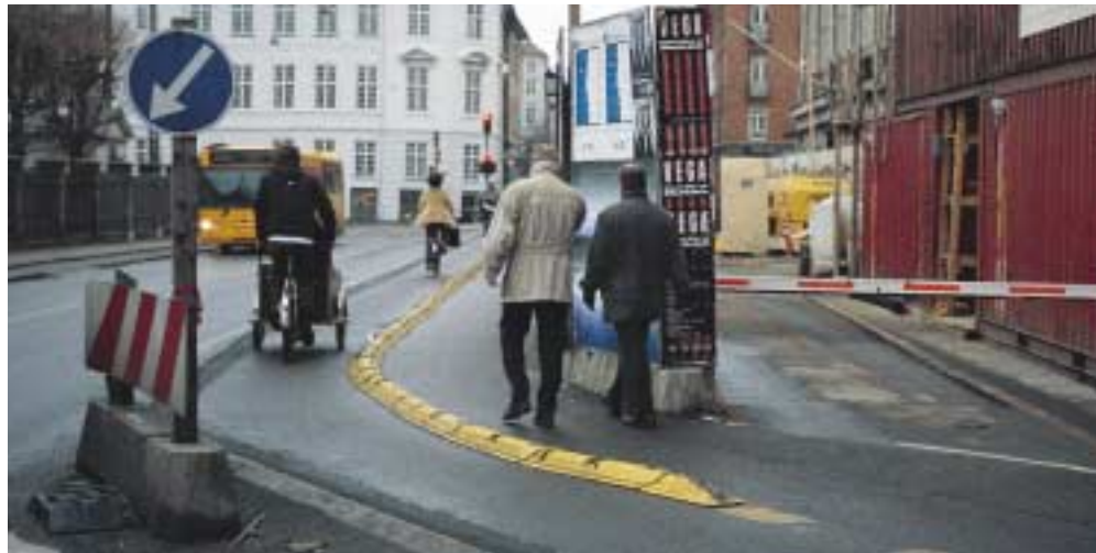
The yellow snake – a good longitudinal guiding barrier.
