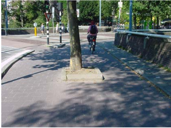
Examples of the introduction of bicycle provisions in the city: The retention of a tree in a bicycle path (Ledig Erf) and the realisation of a bicycle lane (without a legal status) in an inner city regeneration area (Herman Gorterstraat). Note with the latter the parking arrangements.
