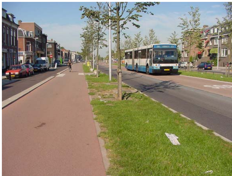
The high-quality public transport lane on the “Vleutenseweg”. One of the sections of the bus lane network that has already been realised. From left to right the photo shows a parallel road, a bicycle path, a grass verge, the main road, the bus lane and the central reservation of the road
