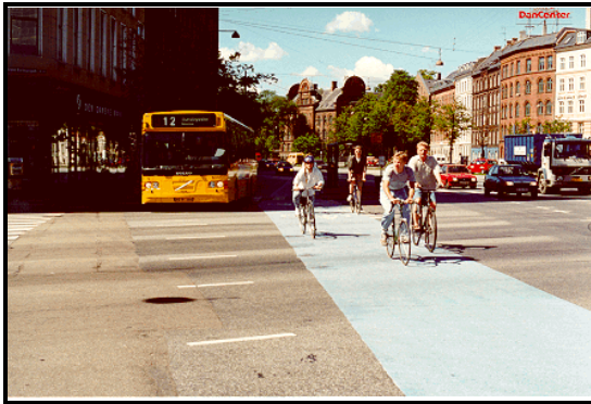
The blue cycle lane continues through the junction as a cycle crossing
