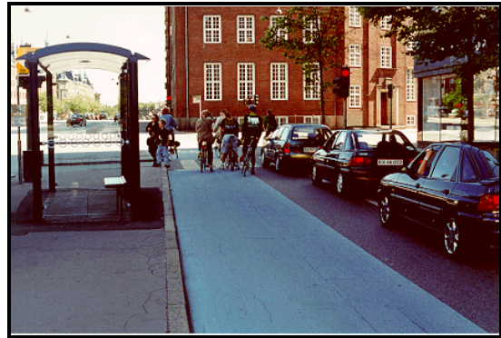
The blue cycle lane between a bus passenger island and the lane for right turning cars
