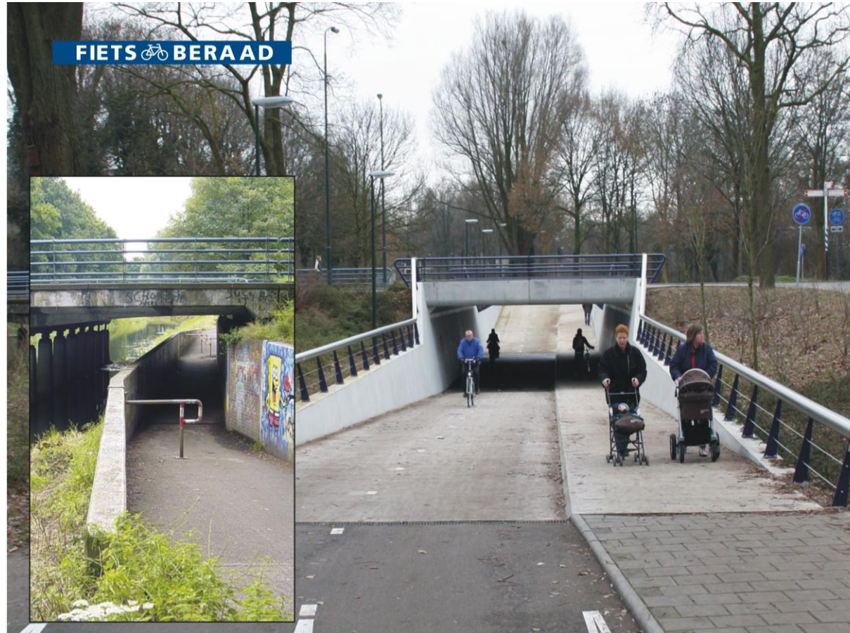
Design-and-construct fietstunnel Veghel, Rembrandttunnel
